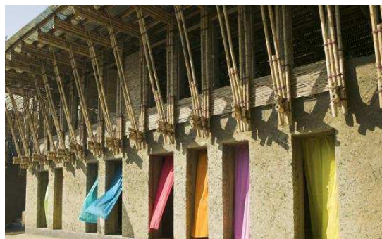
Fig. 3.5.2.1.95. Handmade School, Heringer y Roswag. http://www.worldarchitecture.org/world-buildings/ccfm/meti-handmade-school-in-rudrapur-building-page.html
