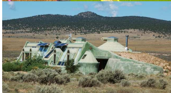
Fig. 3.5.2.1.107. Construcciones Earthships. M. Reynolds. http://kirknelsen.com/project/earthships/
