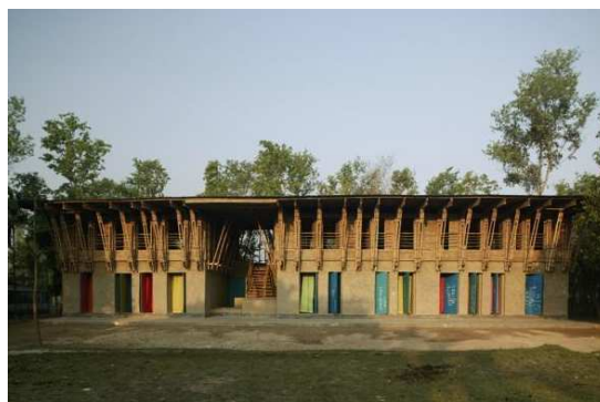
Fig. 3.5.2.1.96. Handmade School, Heringer y Roswag. http://www.worldarchitecture.org/world-buildings/ccfm/meti-handmade-school-in-rudrapur-building-page.html
