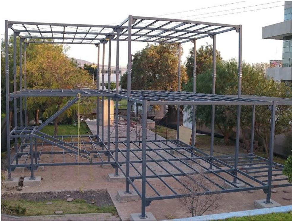
*Figura 5-12. Estructura principal de la “Casa solar experimental”.*
