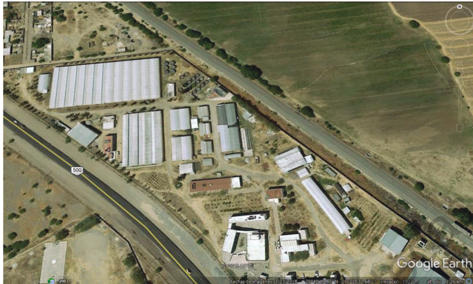
Figura 3. Vista satelital del campus Amazcala (Google Earth, 2018).
