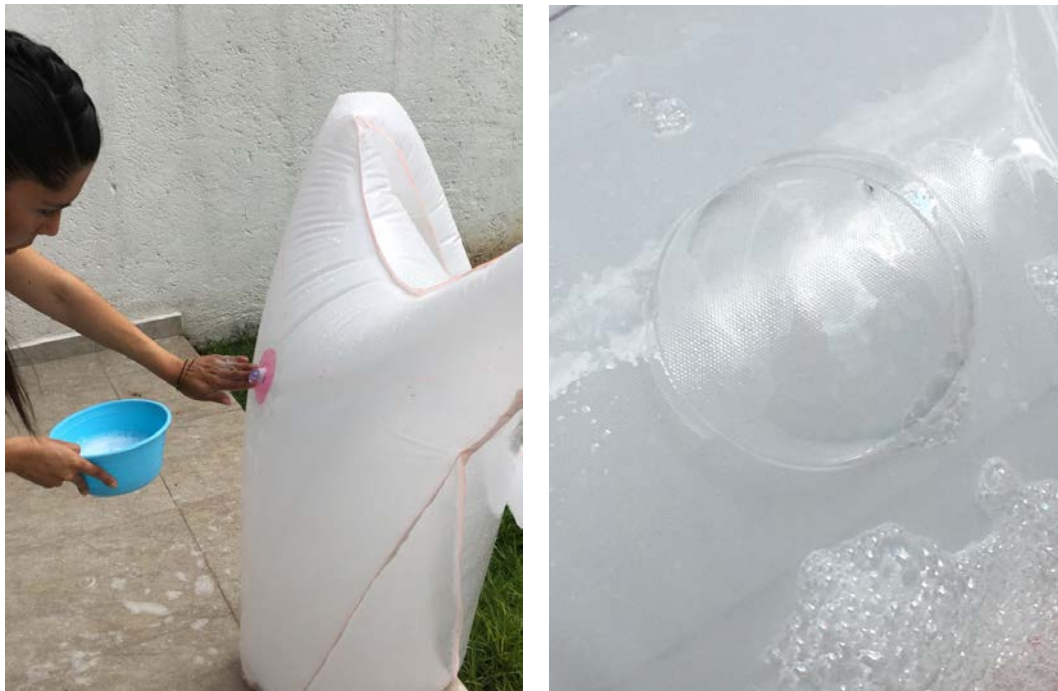
6-50. Perforations repairing process
