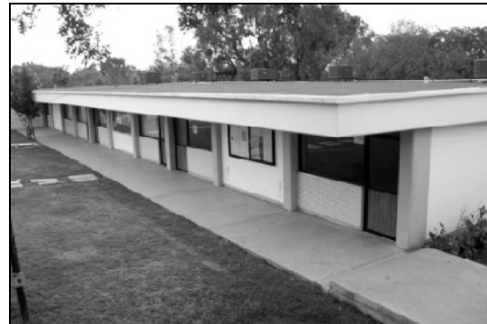
Fig. 3. Building subject to experimentation
