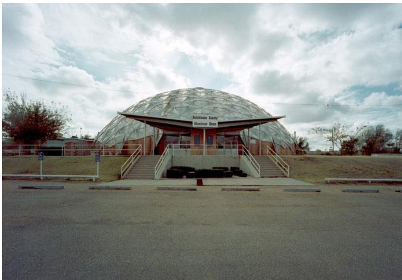
Fig. 2.1 Hutchinson County Aluminum Dome
